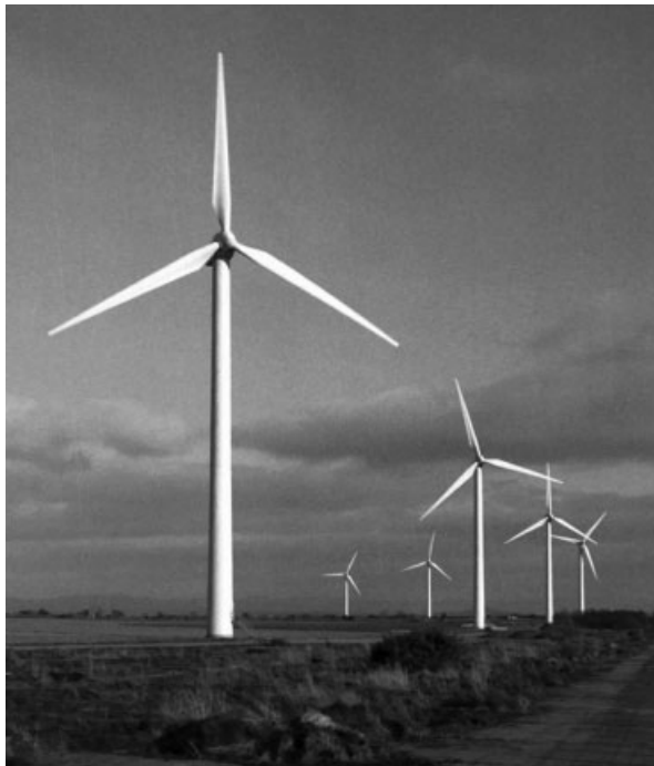
Figure 9.3 Windfarm of Six 660 kW Turbines in Flat Terrain (Reproduced by permission of Cumbria Wind Farms Ltd, Paul Carter)
