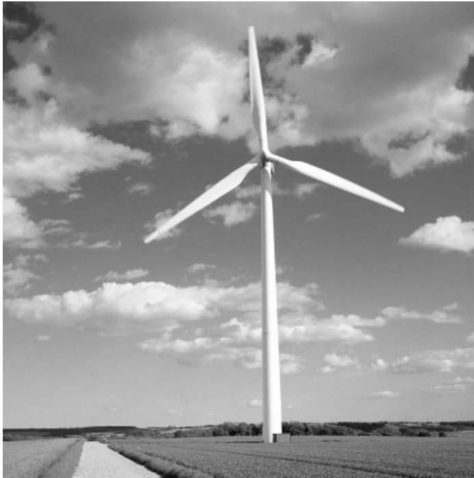
Figure 1.2 750 kW, 48 m diameter Wind Turbine, Denmark (Reproduced by permission of NEG MICON, www.neg-micon.dk )
