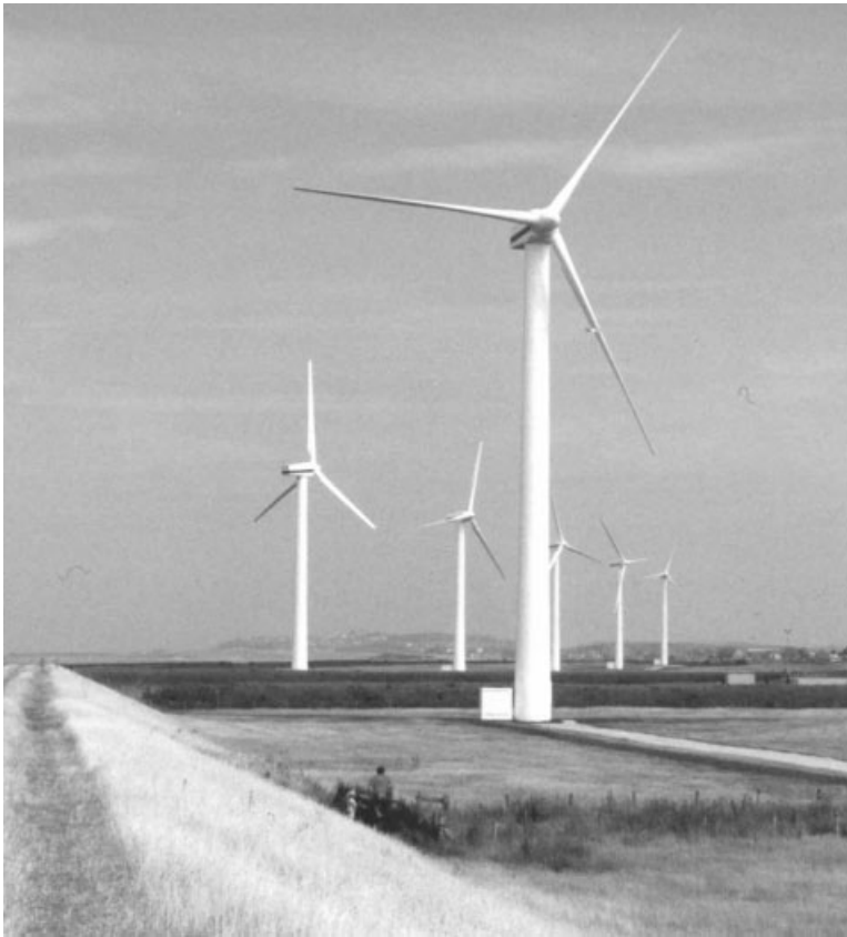
Figure 1.5 Wind Farm of Six Pitch-regulated Wind Turbines in Flat Terrain (Reproduced by permission of Wind Prospect Ltd., www.windprospect.com )
