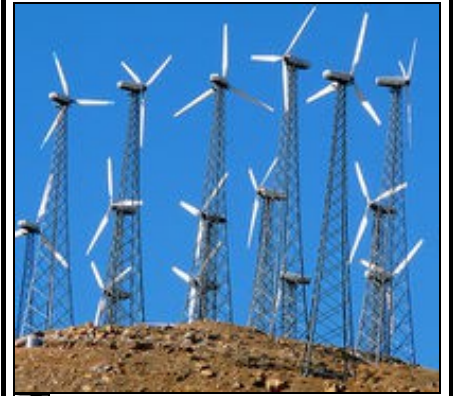
Fig 8(b) Lattice tower
