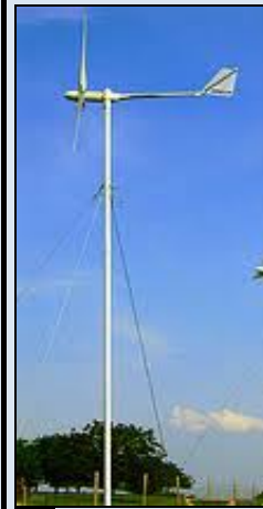
Fig 8(c) Guy tower
