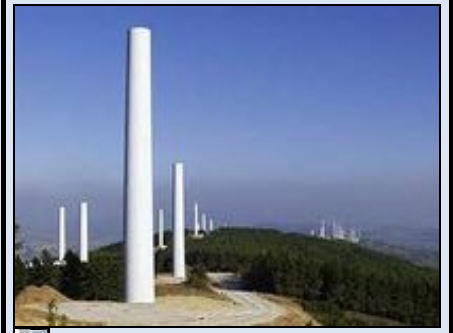
Fig 8(a) Tubular tower
