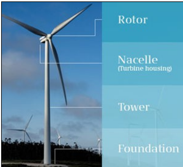
Fig 6 Wind turbine parts
